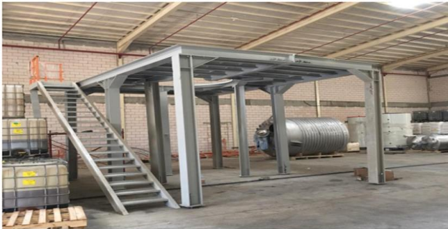
Figure 8: Part of infrastructure inside the factory
