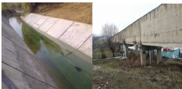
Fig. 6&7, The open canal and aqueducts
