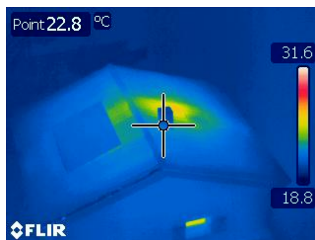
Figure 17: Roof top view with double wall and ceiling insulation
