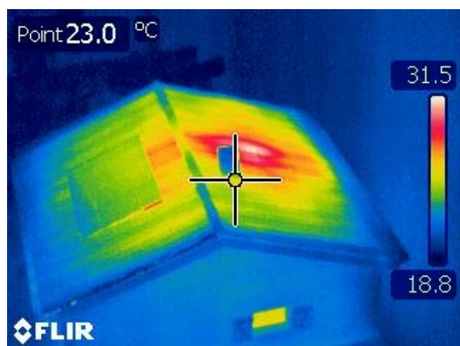
Figure 16: Roof top view without double wall and ceiling insulation
