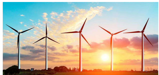
Figure 1: Wind farm onshore (West Baker in Egypt).
