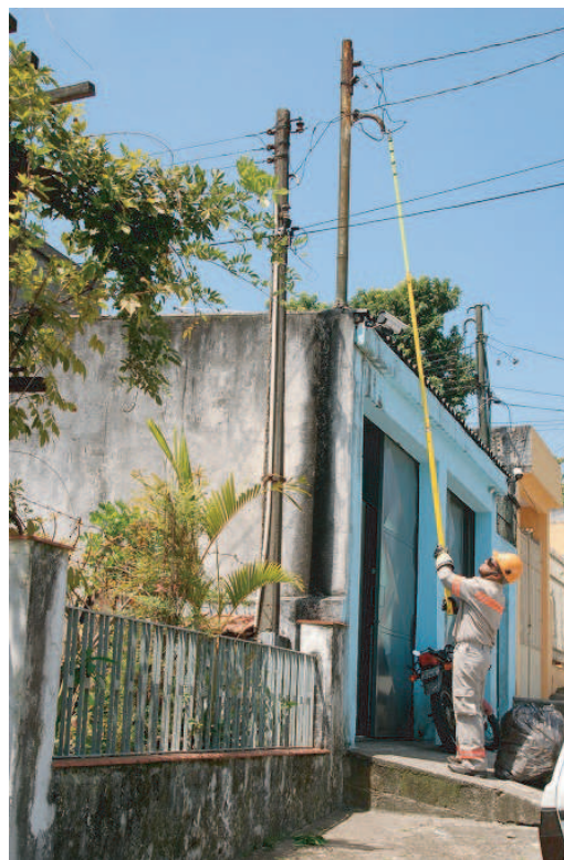
Fig. 3 A linesman installing the electronics device in a wiring connection of AES Eletropaulo.
