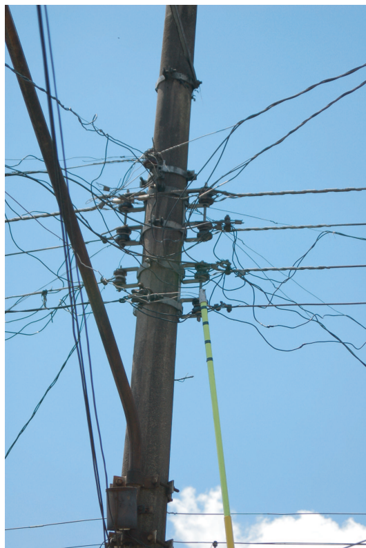
Fig. 4 Wiring of a typical pole connection in a poor region of the AES Eletropaulo concession area in the city of São Paulo.
