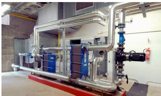
Fig. 6. Heat exchanger station
