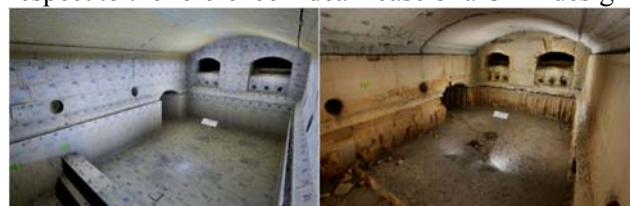
Fig.1. Glass furnace in new conditions (left) and before demolition (right)
