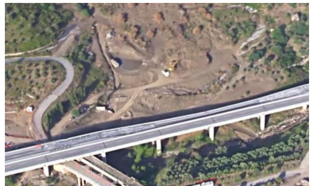
Figure 3 - Landslide close to the HIMERA viaduct.
