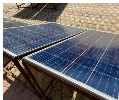
Figure 10: Solar Panel after applying the prepared Nano-coating.
