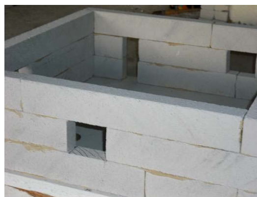
Figure 2: AAC external walls building
