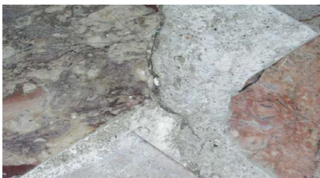
**Figure 11:** Cracking in house floor [Source: Hatzopoulou, 2018 [26], Dakoulas, Thanopoulos, Belesis, Lazaropoulos, 2004 [27]].
