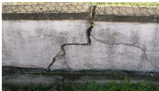
**Figure 14:** Cracking in a courtyard wall. [Source: Hatzopoulou, 2018 [26], Dakoulas, Thanopoulos, Belesis, Lazaropoulos, 2004 [27]]
