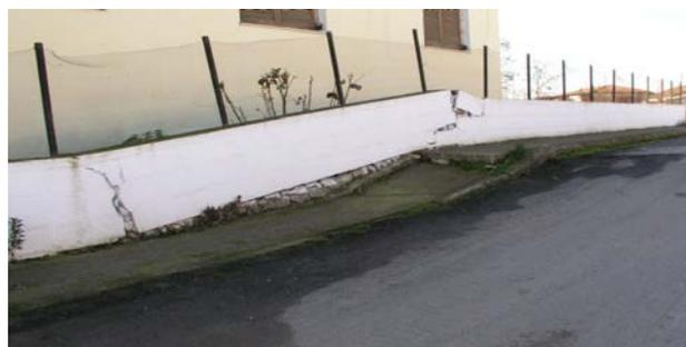
**Figure 15:** Cracking on road surface and a house courtyard [Source: Hatzopoulou, 2018 [26], Dakoulas, Thanopoulos, Belesis, Lazaropoulos, 2004 [27]]
