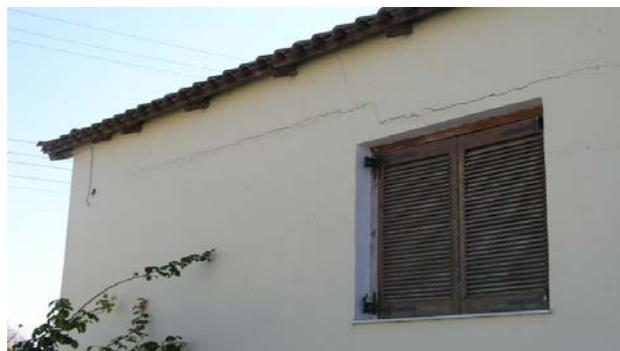
**Figure 9:** Cracks in exterior house wall [Source: Hatzopoulou, 2018 [26], Dakoulas, Thanopoulos, Belesis, Lazaropoulos, 2004 [27]].
