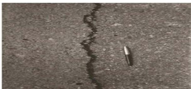
**Figure 8:** 5 mm crack on the asphalt in the Theban field area [Source: Christodoulias and Giannaros, 2018 [24]]
