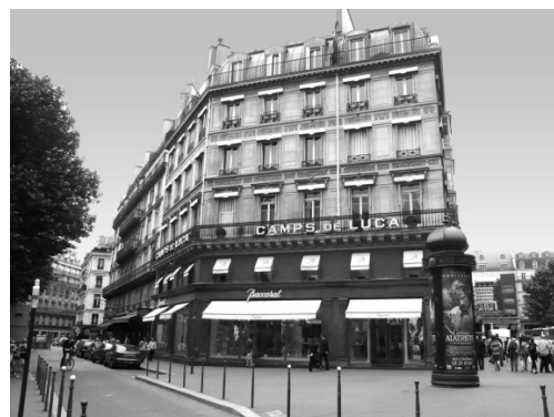
Fig. 2 – Facade front view
