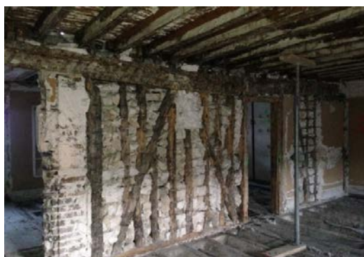
Fig. 6 - Clay bricks infill
