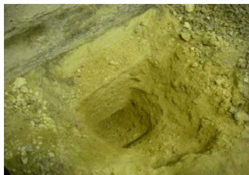
Fig. 17 – Limestone masonry strip footing
