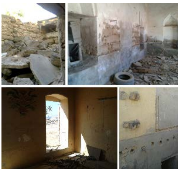
Fig. 3 Dwelling’s interior spaces (photos by the author).
