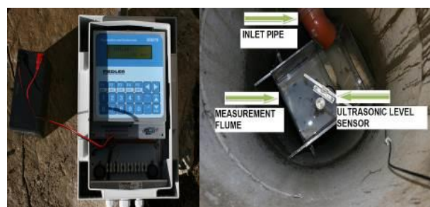
Fig. 7. measurement devices - Data unit M4016 in shaft A, Measurement flume with ultrasonic level sensor
