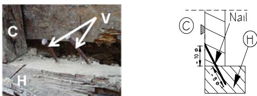
Fig. 20 - Connection between exterior tabique wall and the bottom rails
