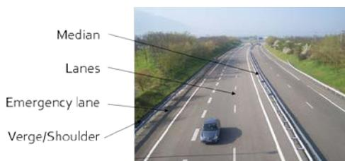
Figure 2 Ribbon model applied to a motorway.
