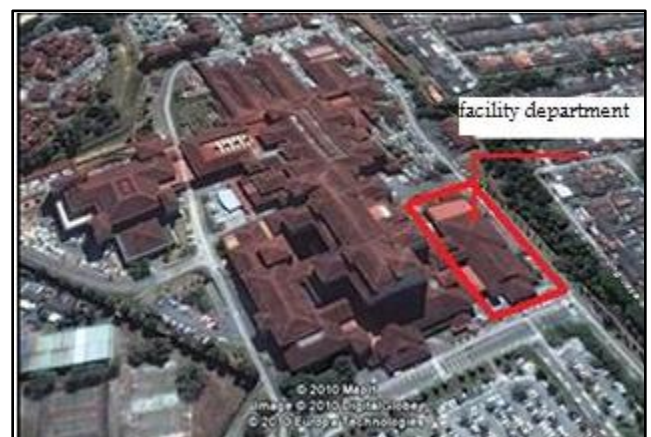
Fig.1: General view of HUKM and Facility department.
