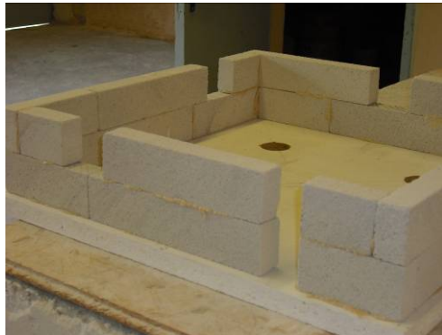
Figure 5: AAC external wall
