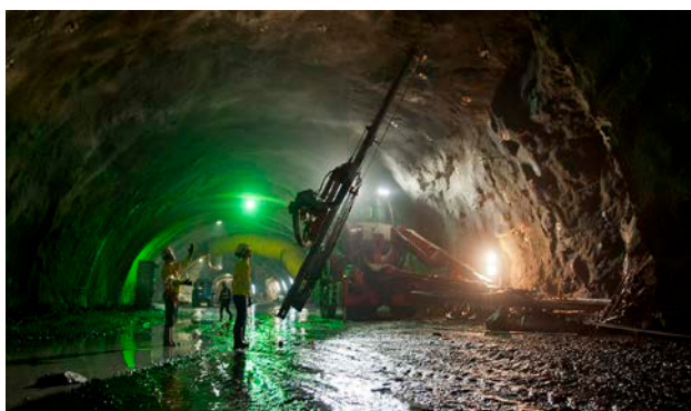
Fig. 1: Complex supporting operation under ground water conditions
