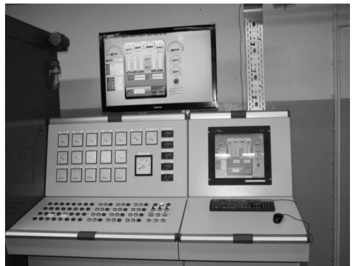
Fig. 2. General view of operating station EMOS
